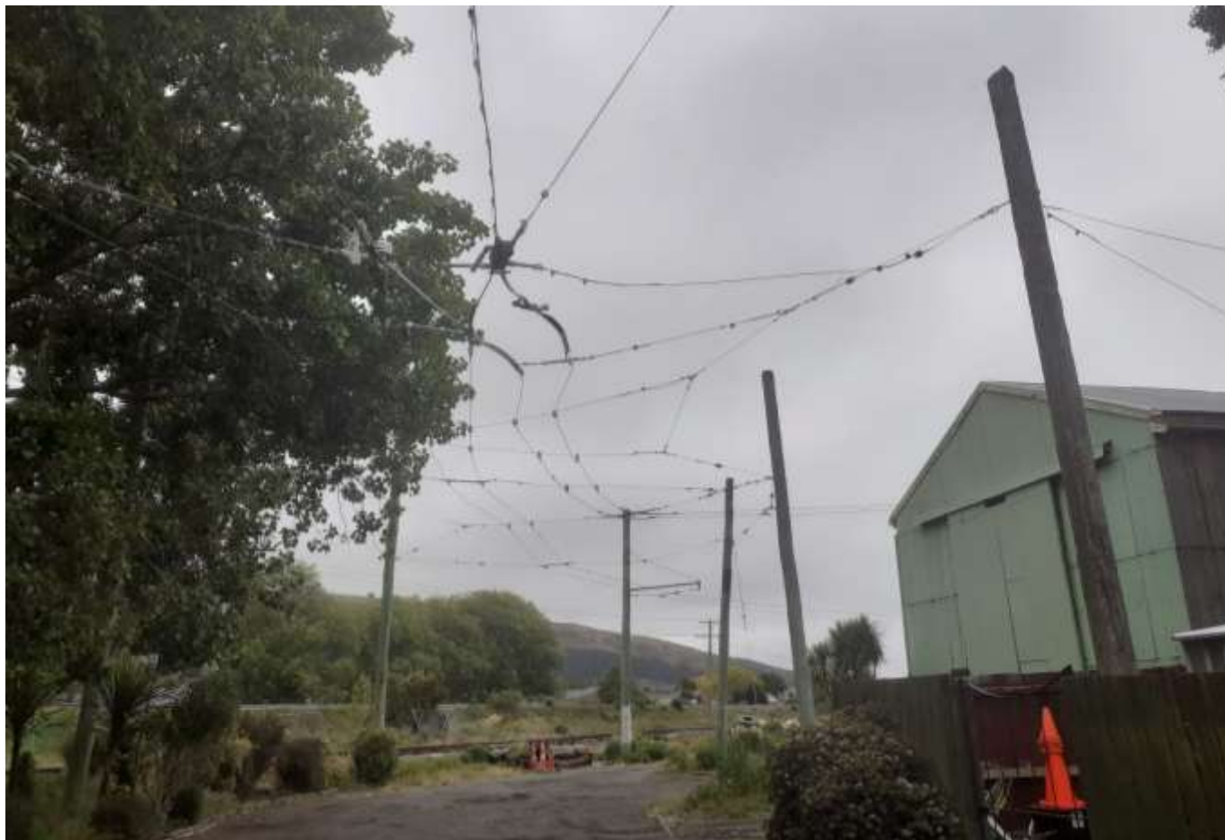
ABOVE: The new right-hand points installed in the overhead behind the Trolleybus Shed. Photo: Alan Roi
