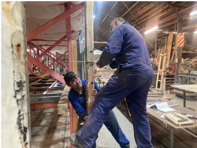
Alan Hinman and Graeme cut through a decayed bulkhead pillar
