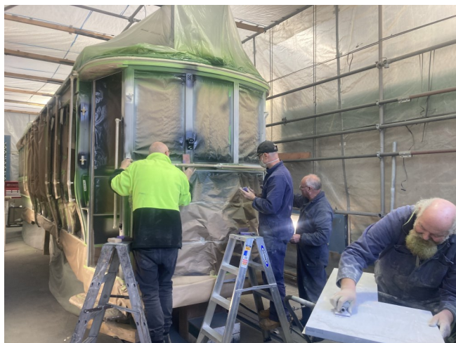
The HTT staff sanding 24 ready for the Cream colour to be applied.
