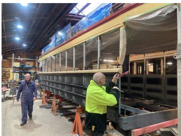
Brian and Warren trial fit the new window sill.
