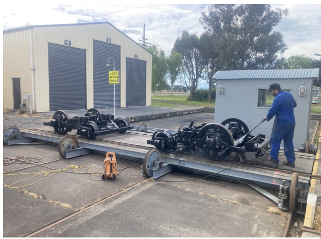
Alan Hinman waterblasting the trucks before painting.
