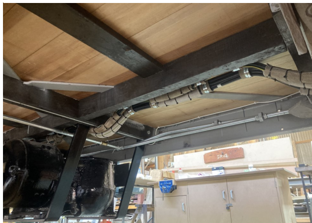
The new piping and wiring in place under the car.
