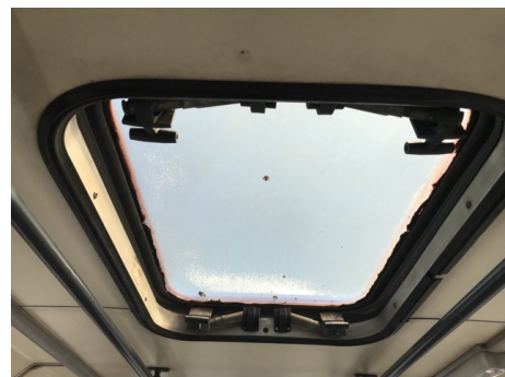
Before the roof window was replaced.
