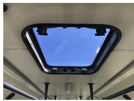
Showing the new roof window in place.
