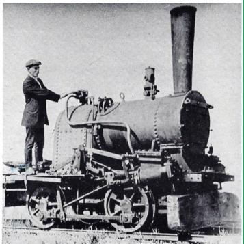
In its original form the Rowan engine was identical to this Kitson steam motor of the Canterbury Tramway Company: in its last years it worked sans cab. G. C. Stewart coll.
